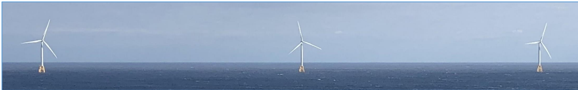
Block Island Wind Farm
